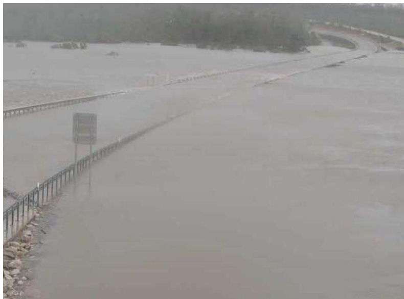
The new bridge over the Archer River was tested. Picture: TMR
