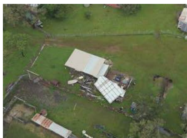
Narelle damage. Picture: QPS
